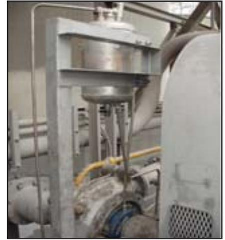
AESSEAL® water management system on slurry pump duty.
