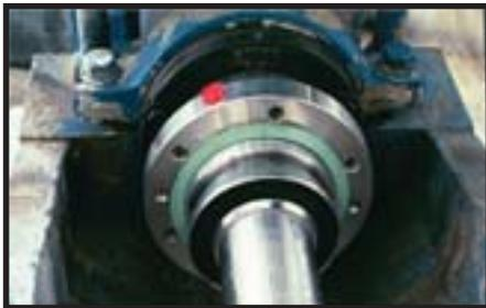
CVSD™ installed on a Slurry pump.
