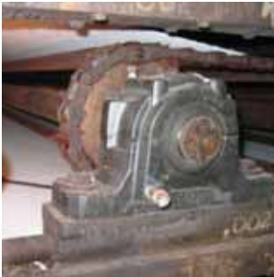
Pulp & Paper Industry, Canada. LabTecta-PB™ installed on a dryer roll (Case Ref: 3369)
